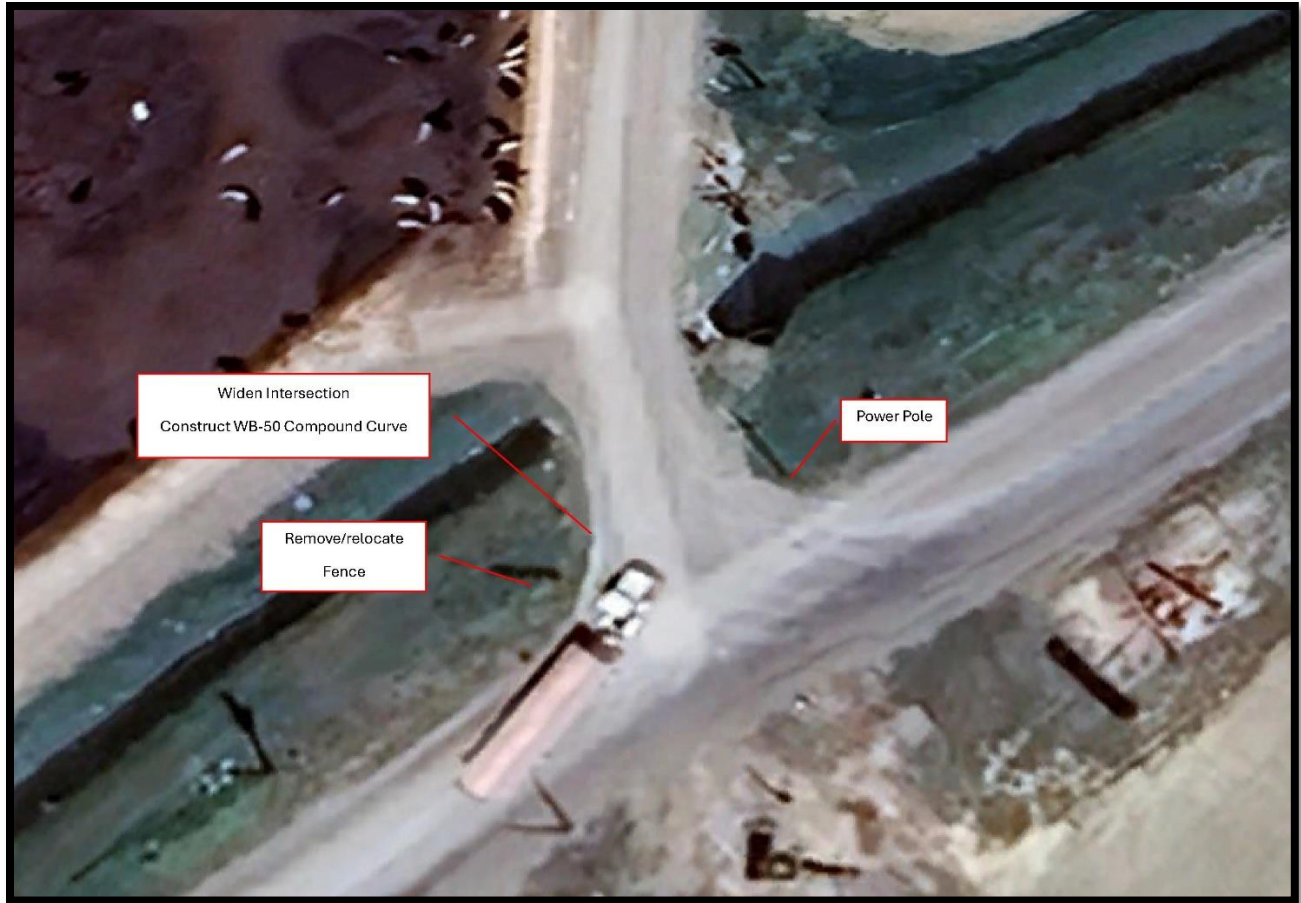
Figure 8: New Access Improvements
